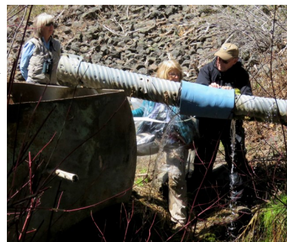
Fixing the water pipe at Reecer. (C. Clark)
